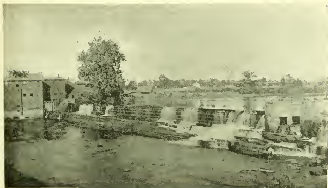
A View of the Dam—Chicopee Falls
